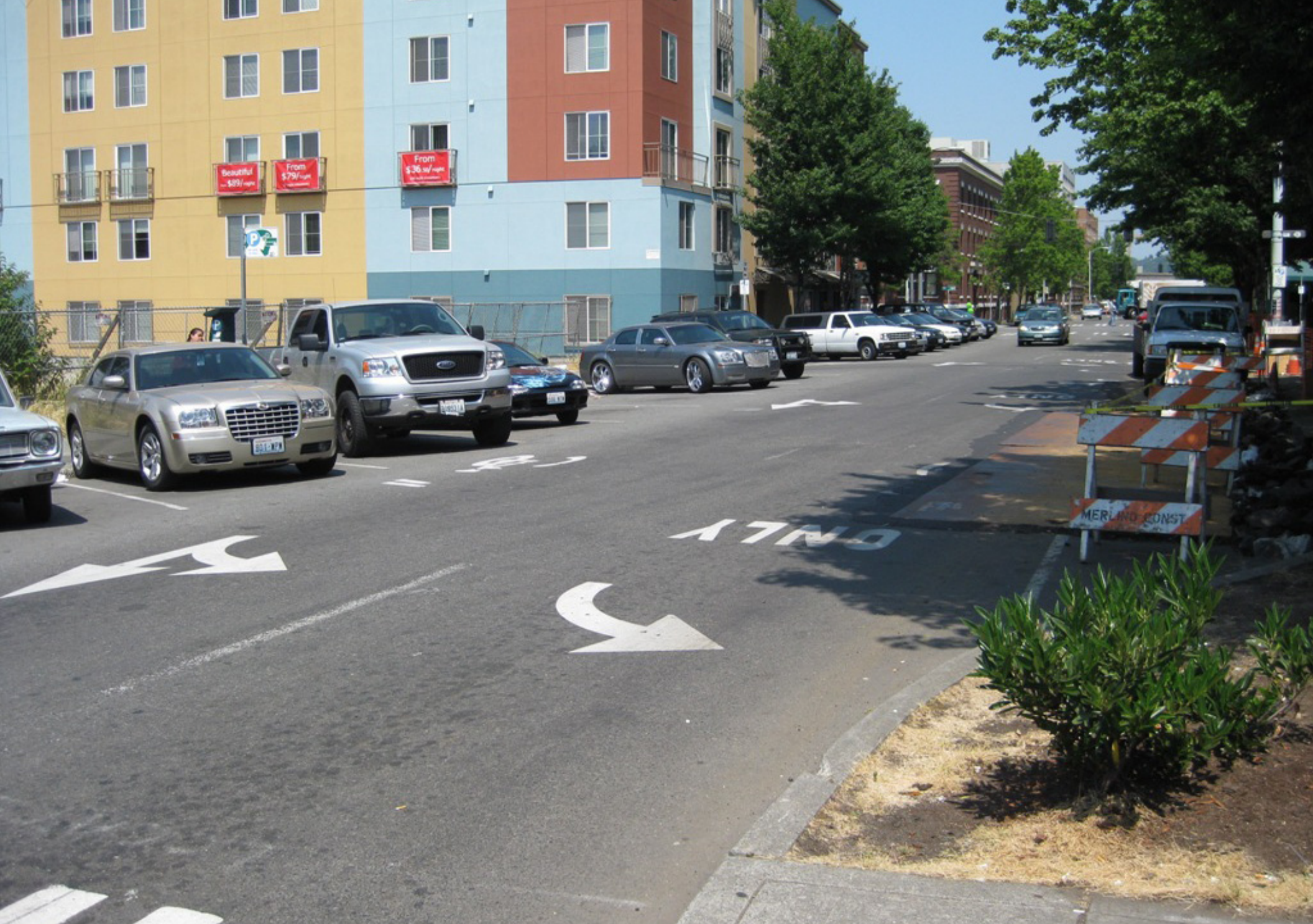
02. Prior to construction, Bell Street was composed of two westbound vehicular lanes flanked by parking and narrow crumbling sidewalks on either side. Storefronts were vacant, walking and biking were poorly accommodated and neighbors were concerned about rising crime.
