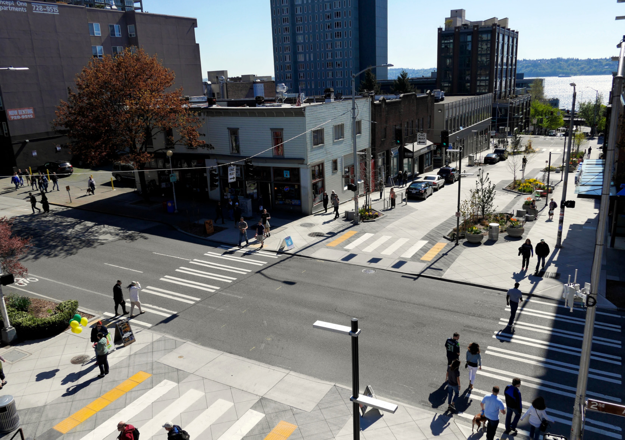
03. After construction, Bell Street Park is a curbsless shared space with slower vehicular speeds and abundant street life. New businesses are open, sidewalk cafes are full and the diverse residents of Belltown have a shared outdoor living room.
